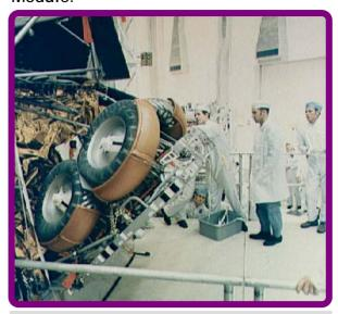
The Lunar Roving Vehicle folded and ready to be inserted into its wedge-shaped stowage compartment
